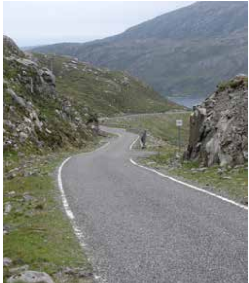
Part of the Rhenigidale road, when completed.
