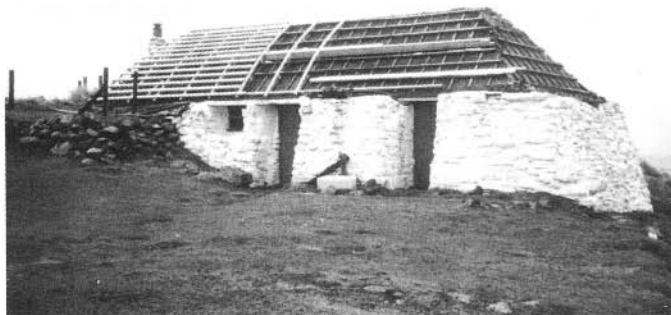
The curved timbers being applied to the roof. April 2002. (Photo: Lawrence Washington)
